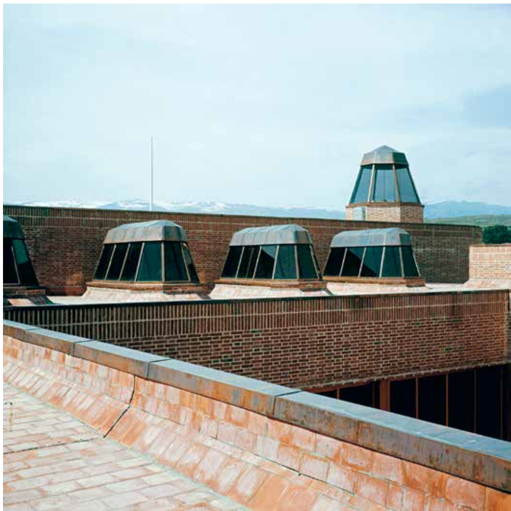
View of the courtyard roofs with the skylights. Vista de las cubiertas del claustro.
